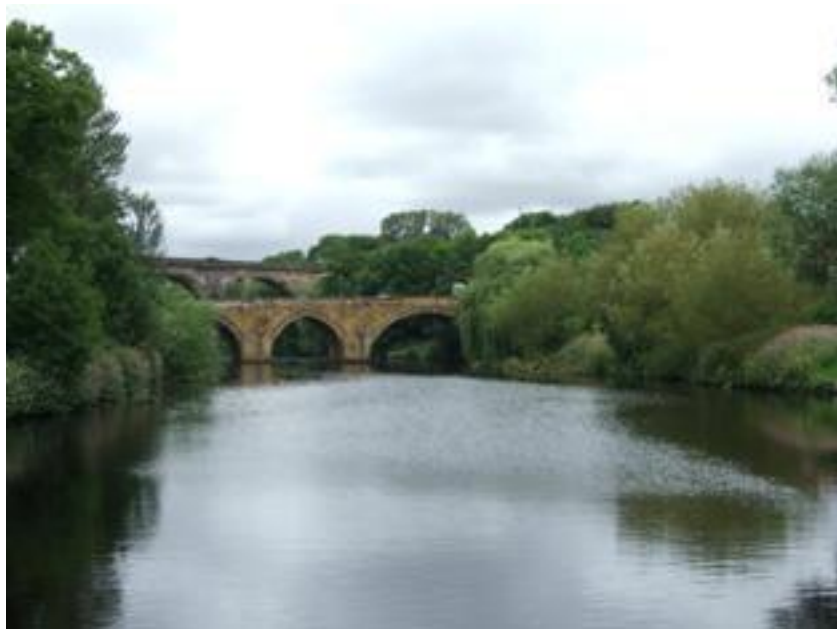
The Two Bridges. Yarm.
